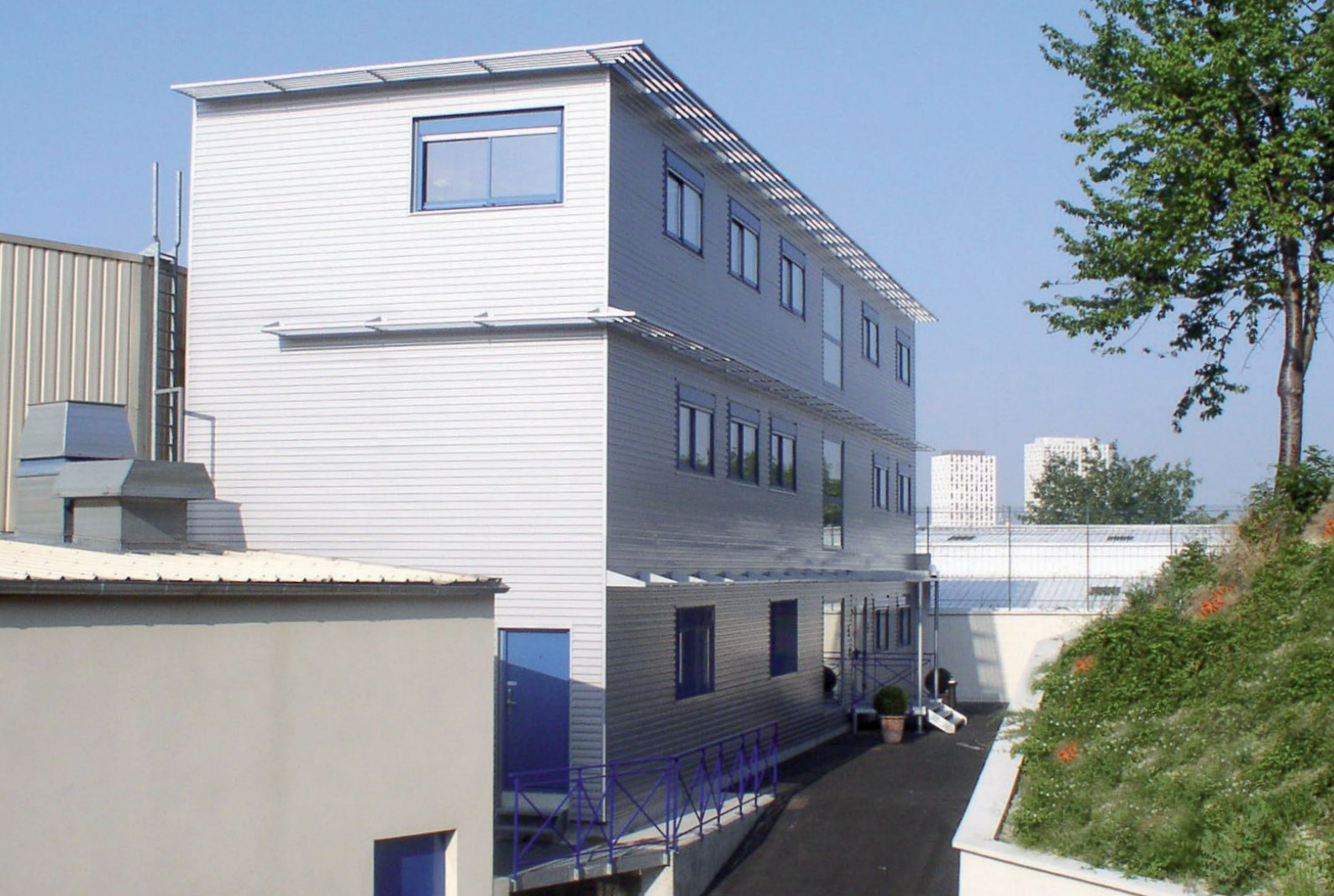
Facility in BAGNOLET
