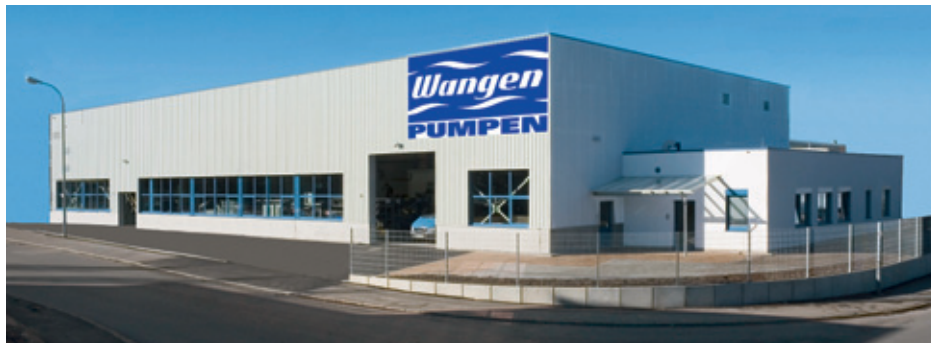
Stator factory at Wangen headquarters
